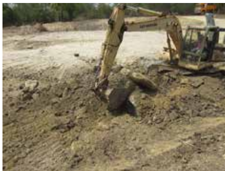
The second pond had a few surprises; one of them was a solid layer of lime stone which was quite a challenge for the excavator.
