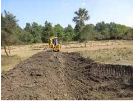
The excavator dug 688 hours to complete the job.
